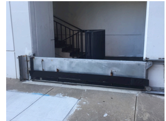
Installed to protect underground spaces
