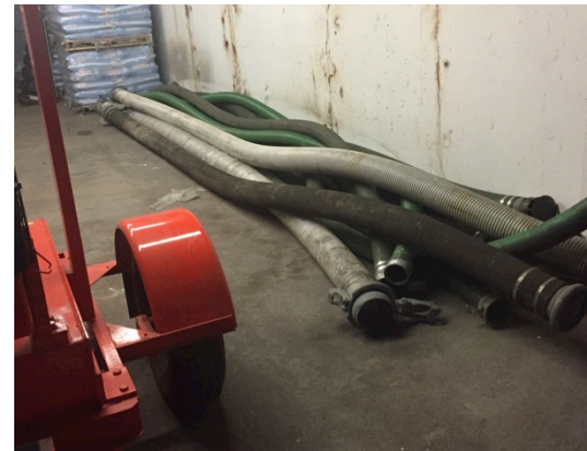
Previously installed pumps ran full time as needed
